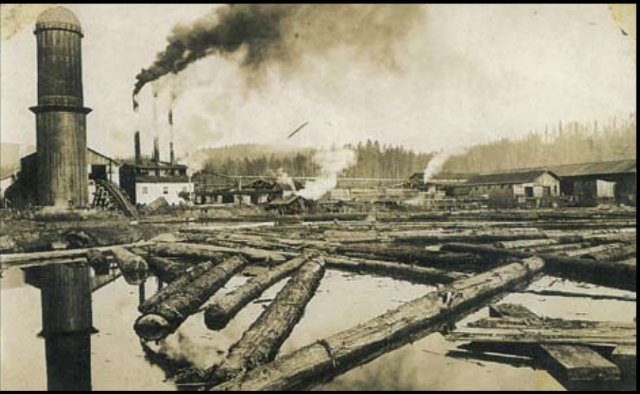
The mill pond with the burner and boiler room behind
